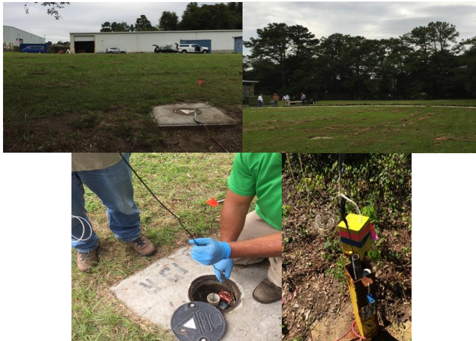
Figure 2.1: (Clockwise from top right) Site preparation and laying out conduit for wire protection; installation of an electrode in hill-side wells; installation of electrode in primary site area; warehouse sheltering low-intensity power source.
